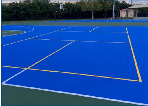
Vizcaya Park Basketball Court Resurfacing
