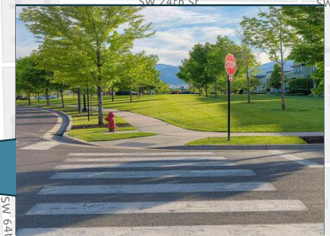
New Sidewalk Connections
